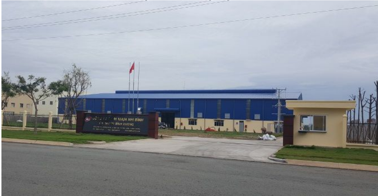
Factory 3,500 m2 in land 10,000m2 at VSIP II, Binh Duong Province
